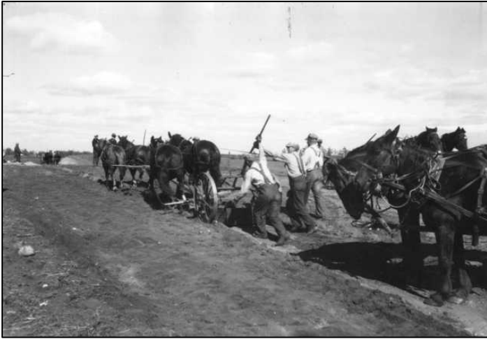
Federal Emergency Relief Administration farm to market road construction project near Alexandria, MN, 1936.
